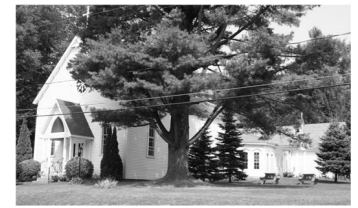
St. Paul's 771 Route 29, Rock City Falls
